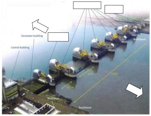
In non-flood conditions, the gates lie flat on the river bed, allowing free passage of river traffic.
