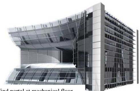
Wind portal at mechanical floor
